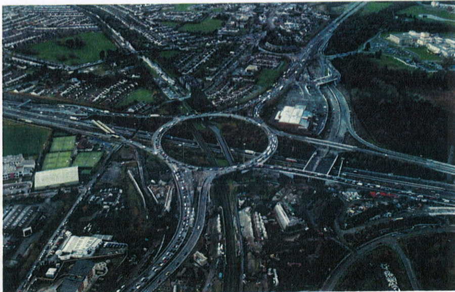
The M50/N3 interchange: A viaduct is being built (bottom of picture) where a tunnel was planned
