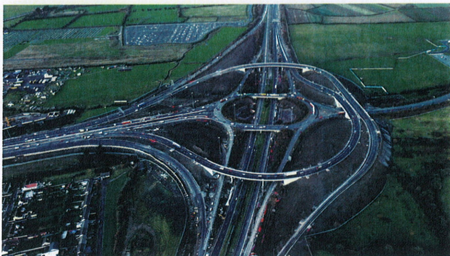
The newly expanded M50/M1 interchange: Curved steel composite structures carry new free flow links
