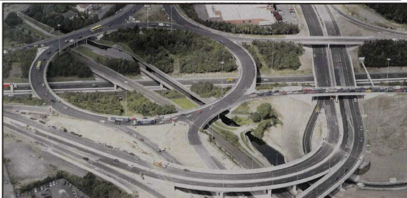
The M50 upgrade PPP Scheme by ATKINS Ireland: undertaking the works on a live motorway represented an enormous challenge
